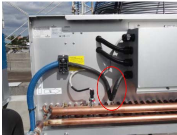
Figure 2-36 Condenser Wiring
