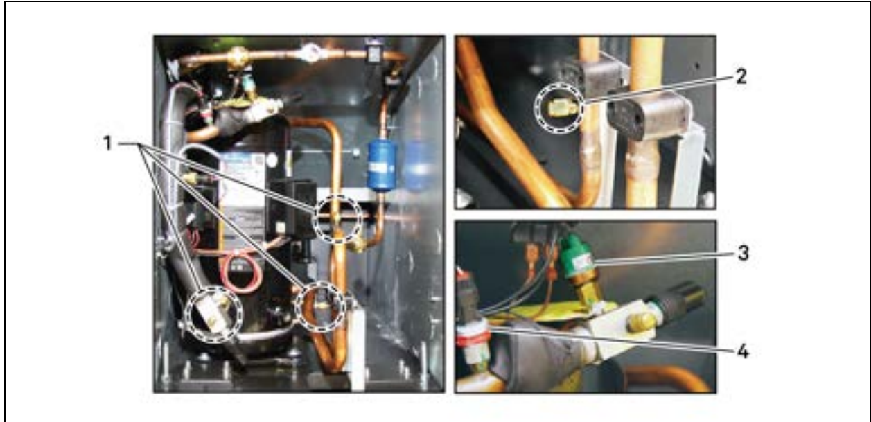
Figure 6.13 Connections for Vacuum Creation and Refrigerant Charge—Air Cooled, 600°mm (24°in.)
