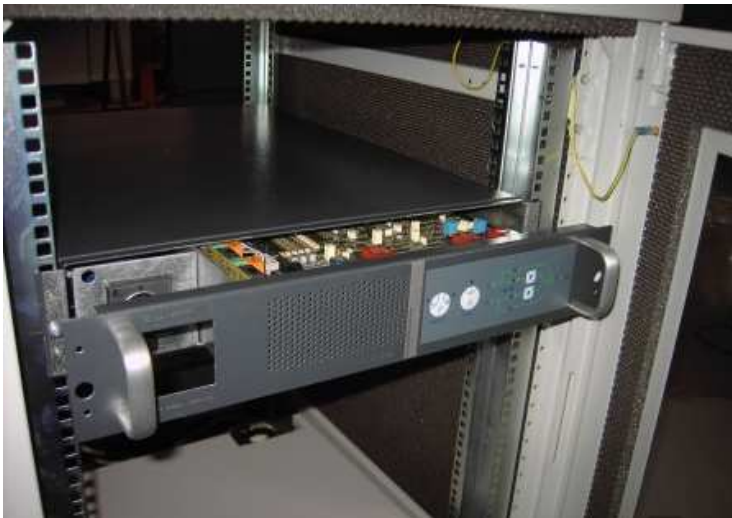
Fig. 13 – Removing the static module
