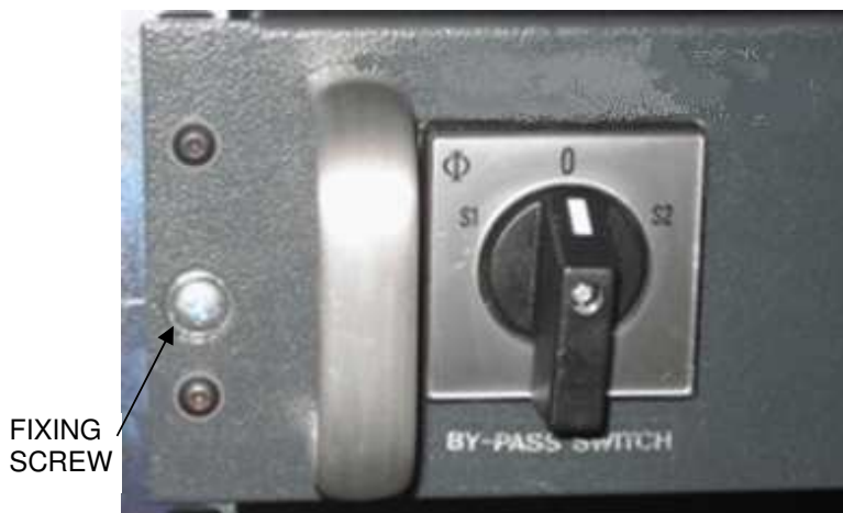
Fig. 7 – Securing Liebert CROSS RACK to the chassis
