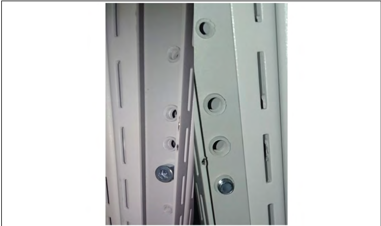
Figure 4.5 Connection of Frame
