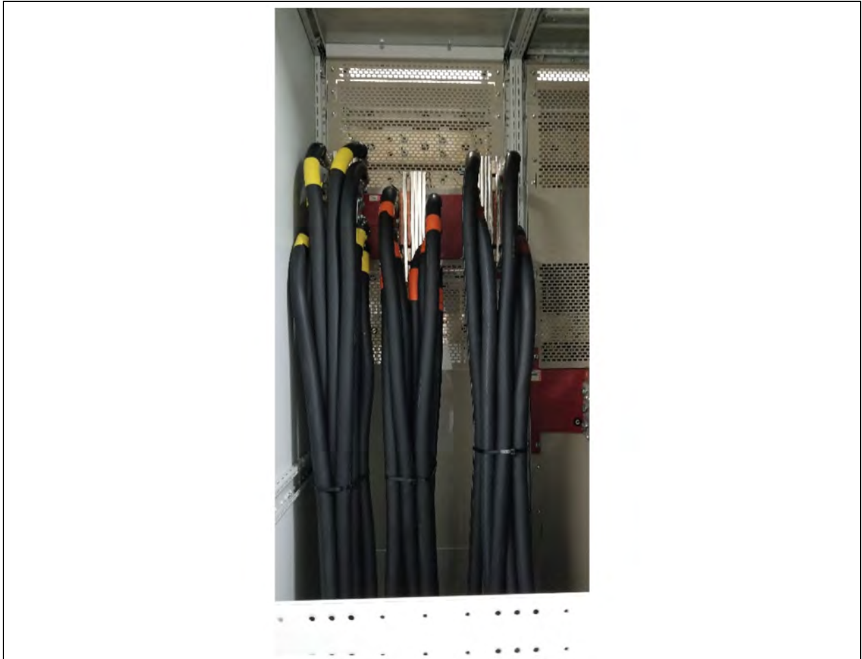
Figure 4.7 Terminated Cables
