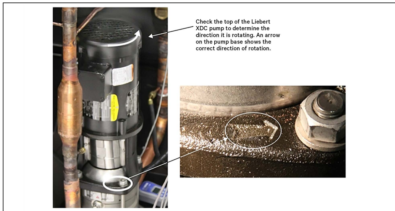
Figure 7.1 Liebert® XDC Pump Rotation Determination
