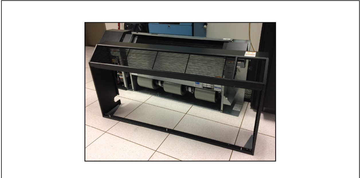
Figure 4.3 Remove Evaporator Panel Assembly
