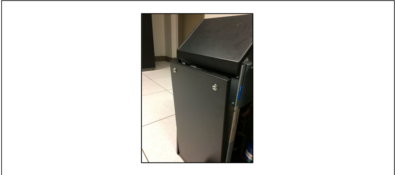
Figure 4.7 Remove Front Access Panel from Condensing Unit
