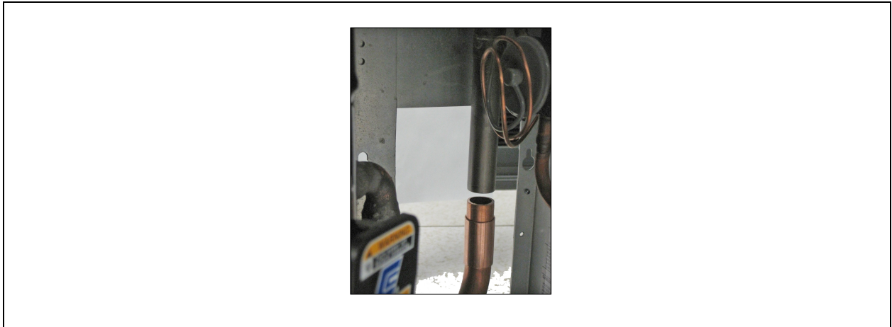
Figure 4.9 Pipe Cut with Tubing Sleeve Installed
