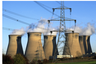
Power plant & Transmission
