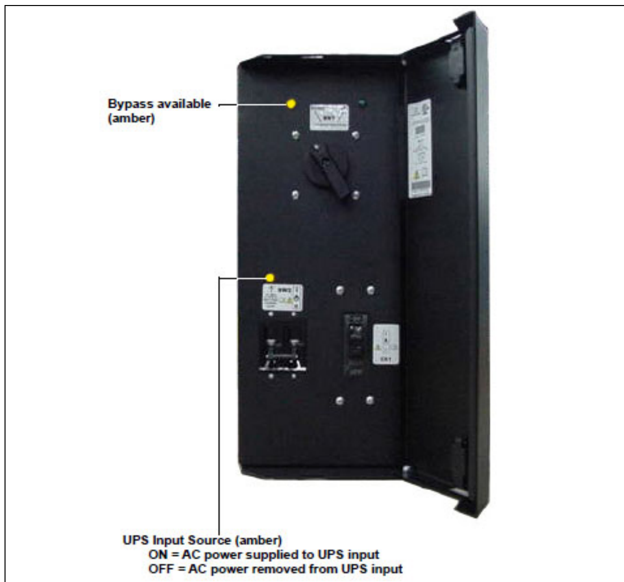
Figure 3.2 Maintenance Bypass Cabinet in Bypass Mode
