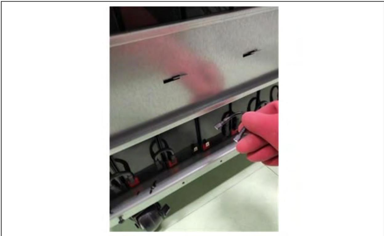
**!** **WARNING!** To perform the servicing UPS, make sure to disconnect the cable connections between the UPS and batteries. Failure to do so may result in electric shock or battery arc risk.
