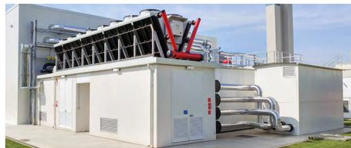
This latest designed lab can test units with cooling capacities up to 1.5 MW with state-of-the-art accuracy in a broad range of working conditions, from -10°C to +55°C, also for adiabatic units.
