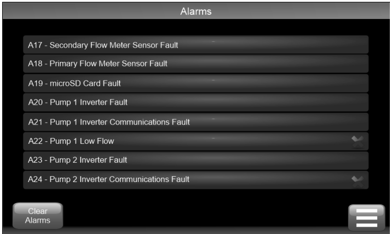
Figure 4.20 Control Screen Alarm Identification
