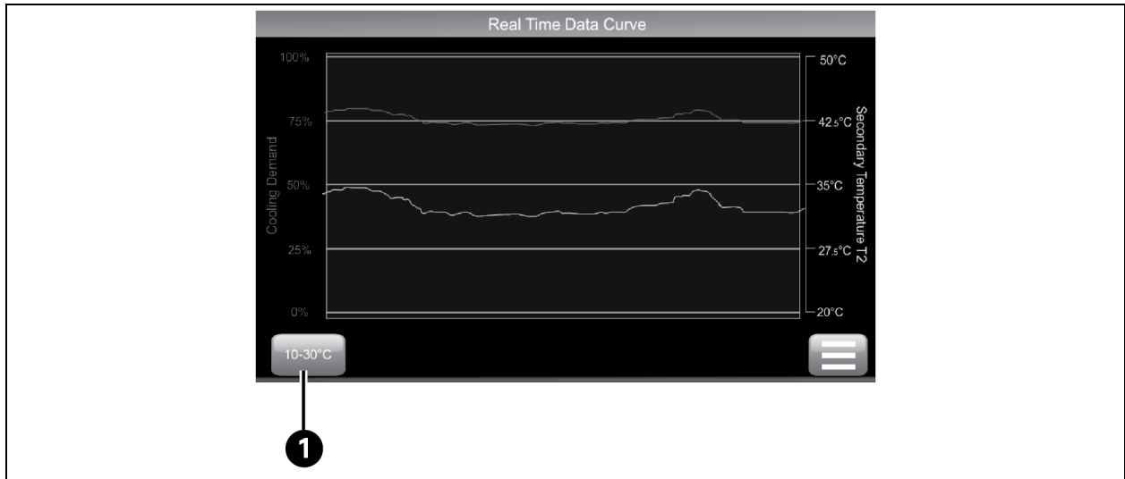
Figure 4.4 Control System Data Curves Screen
