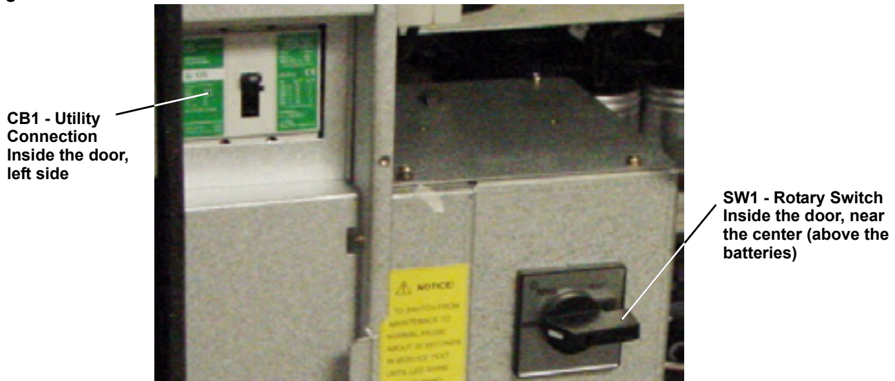
Figure 58 Power switches - 10kVA NX
