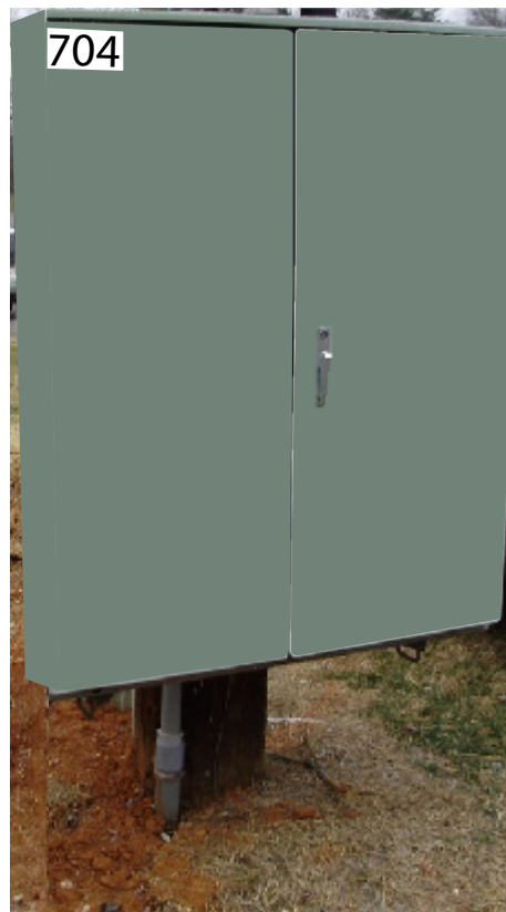
Figure 3: Sample of a host Cross-Connect cabinet
